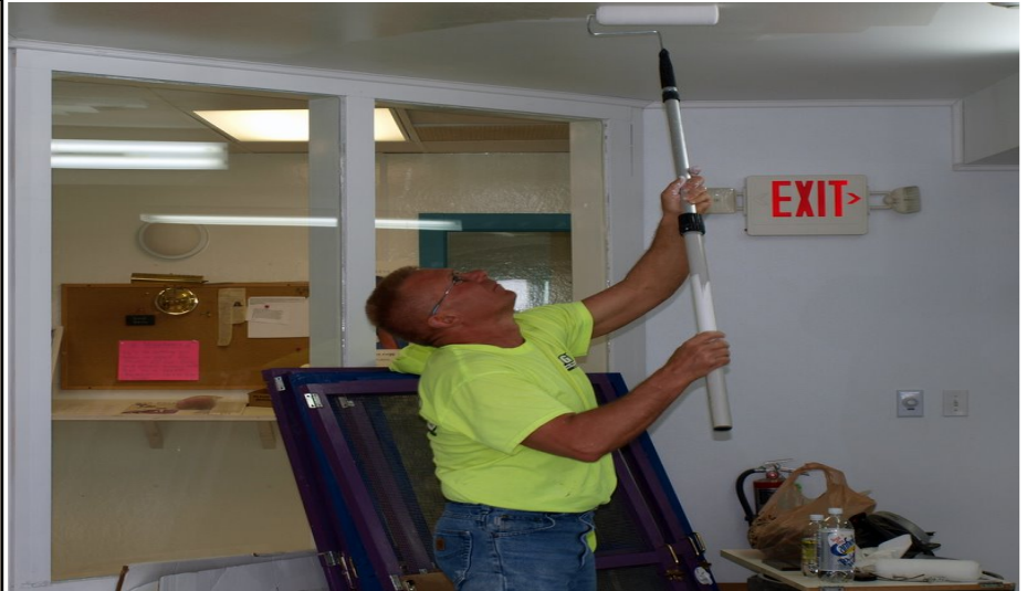
Volunteer Rich Swanson paints the cat room's ceiling.
